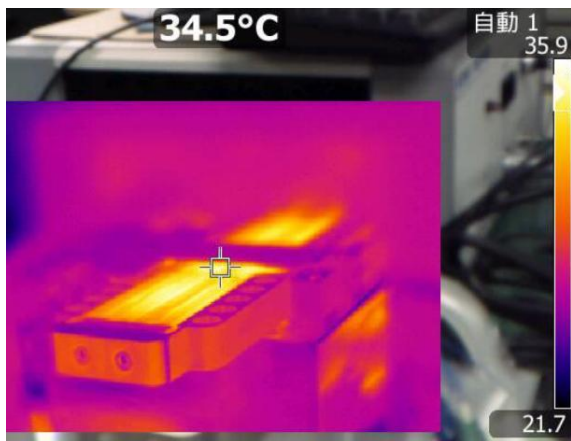
Fig. 7: Thermograph of actuator system
